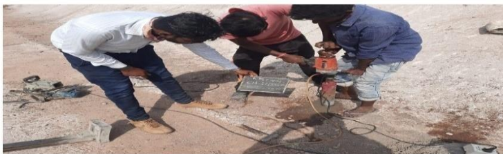
Core Cutting of Arewadi Canal
